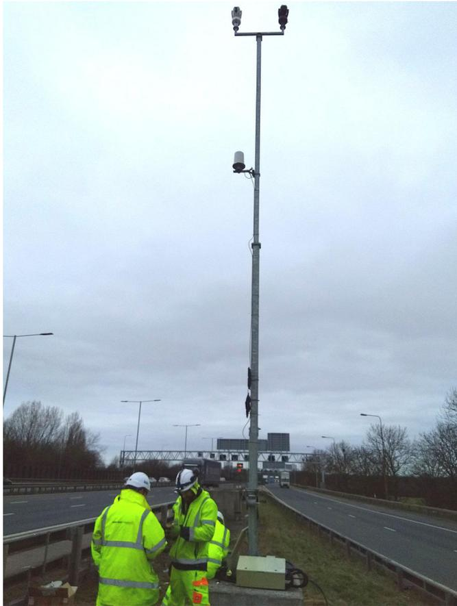
Radar was mounted very high to improve coverage by eliminating obscuration by high-sided vehicles.
